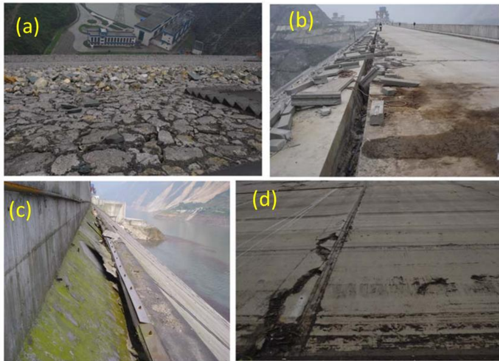
Fig. 11 Earthquake damages to the project structures. (a) loosen rock fills on the downstream side of the dam; (b) open and dislocation of the downstream border of the dam crest; (c) damages of the horizontal joints at the dam crest resulting from subsidence of the wave wall; (d) squeezing damages between the no. 23 and no. 24 slabs.
