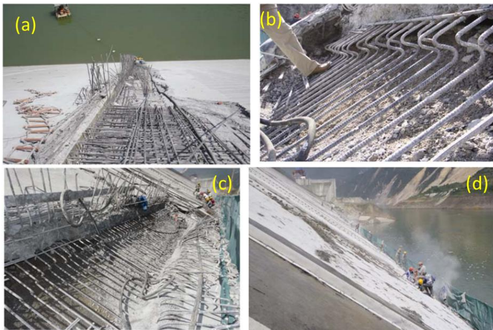
Fig. 12 Dislocation of the horizontal construction joints of the slabs. (a) excavation of the damaged longitudinal joint of the no. 23 slab (after removal of the broken concrete). (b) the exposed horizontal joints at el. 845 m after local removal of concrete. (c) repairing the dislocated horizontal joints of the no.8 slab (the stress bar bended in “s” shape). (d) repairing construction of the damaged slabs.
