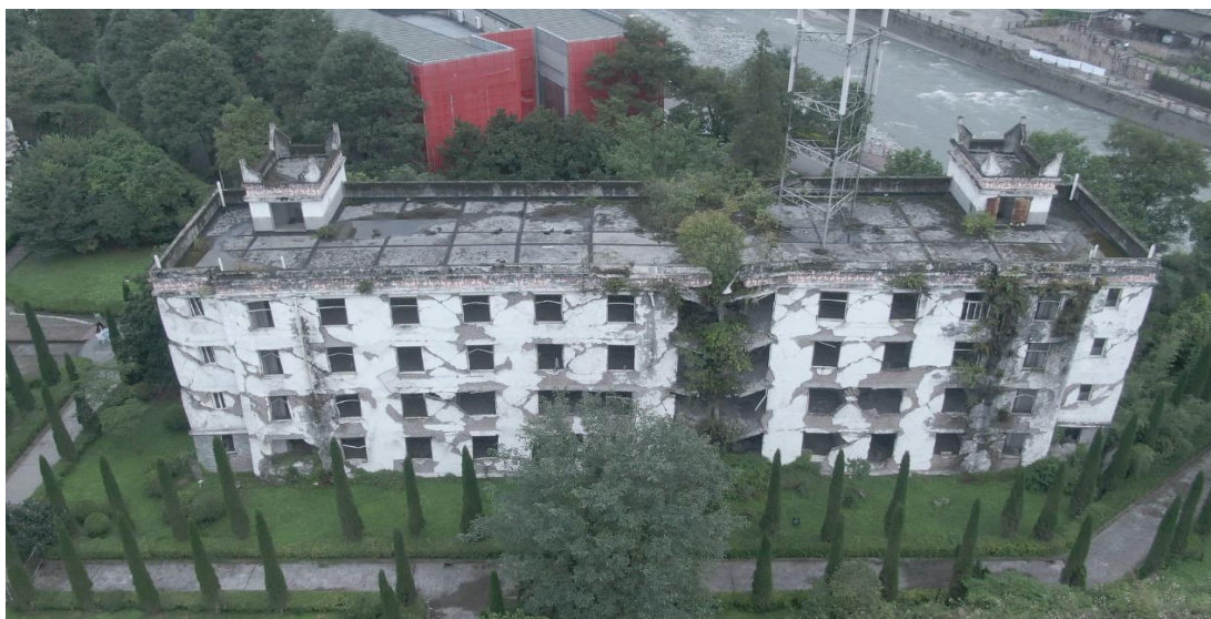
Fig. 17 The earthquake damage of xuankou middle school students' dormitory
