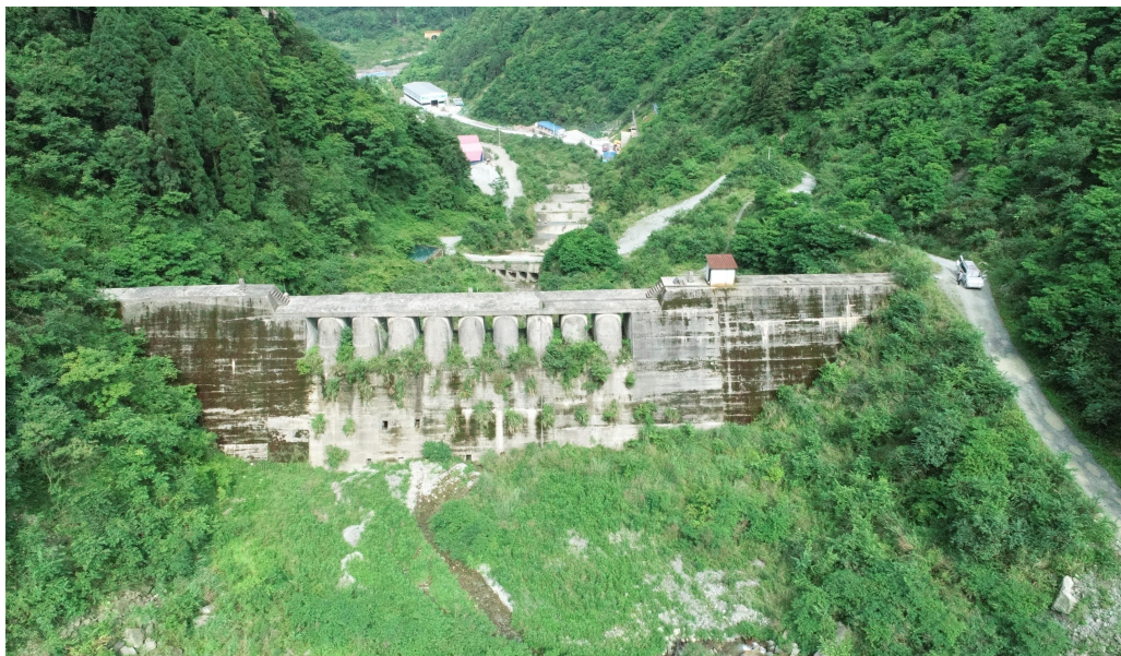
Fig. 24 Check dams constructed in the gully for debris-flow hazard mitigation
