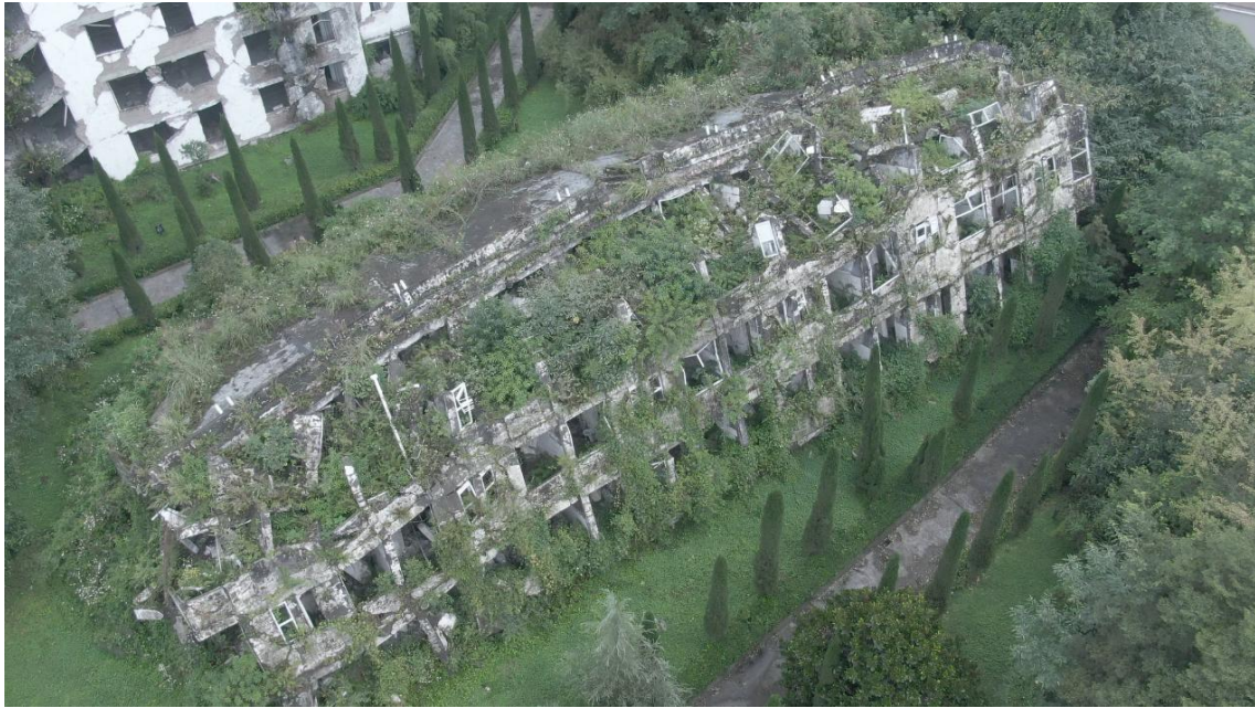
Fig. 18 The earthquake damage of xuankou middle school teaching building
